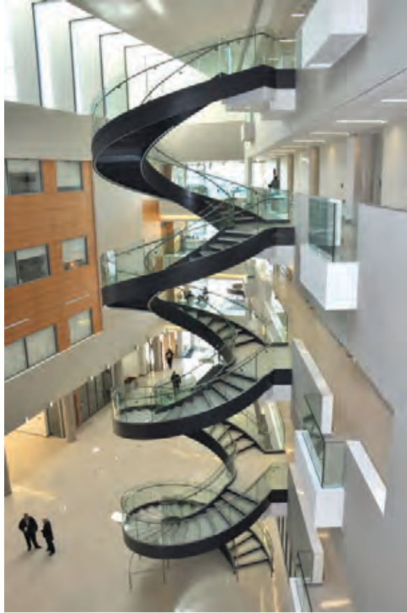
Fig. 1-10. Spiral staircase (courtesy of AISC Bender/Roller Committee).
