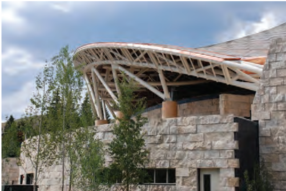
Fig. 1-7. Elliptically curved roof members (courtesy of AISC Bender/Roller Committee).
