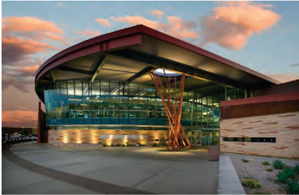
Fig. 1-4. Horizontally curved roof beams for a recreation center (courtesy of AISC Bender/Roller Committee).
