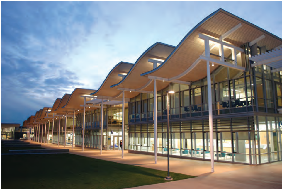
Fig. 1-9. S-shape canopy members (courtesy of AISC Bender/Roller Committee).
