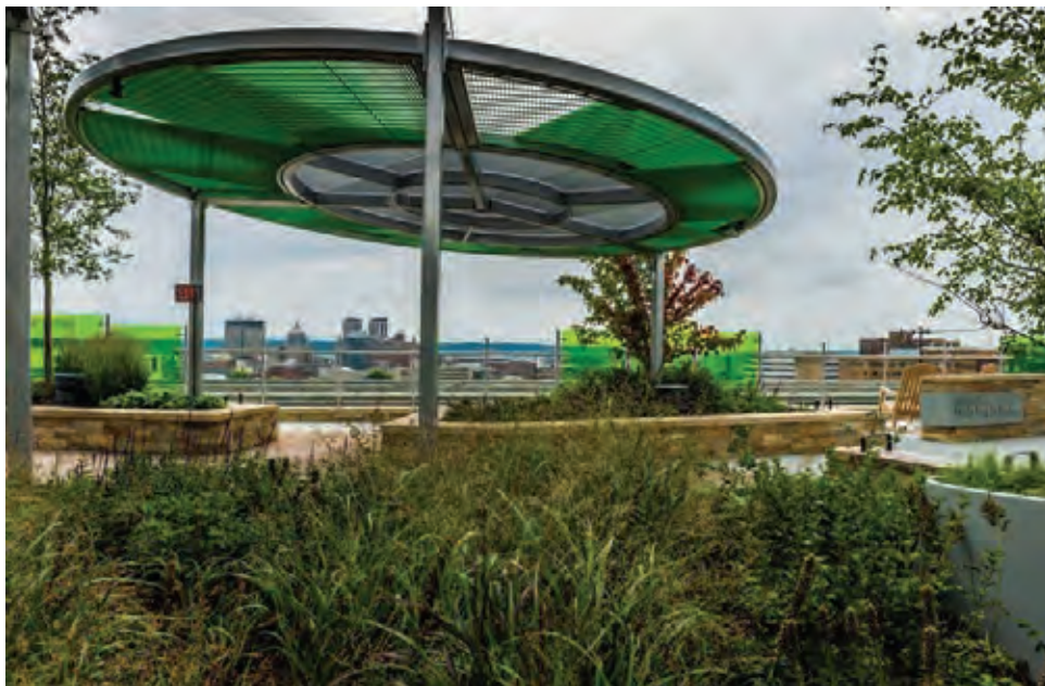
Fig. 1-5. Horizontally curved members for a circular canopy (courtesy of AISC Bender/Roller Committee).
